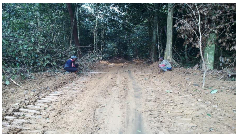
Figure 3: Measuring the width of a skid trail
